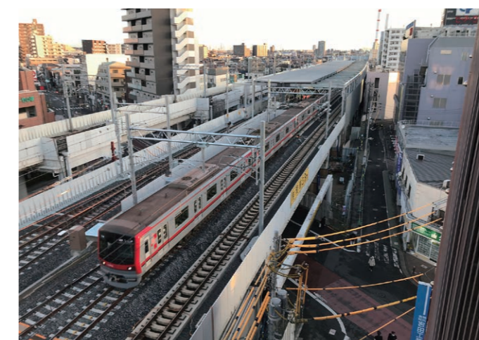
Elevation project in area around Tokyo Skytree Station
